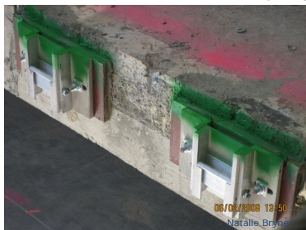
Figure 23: Curtainwall panel's anchors
