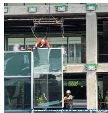
Figure 21: Photograph showing the installation of a curtain wall panel
